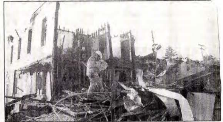
Fire destroys McIntyre Hotel 2004
