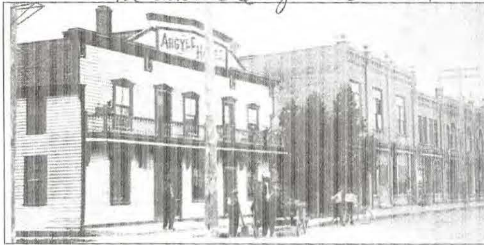
Argyle House 1870s-1961, West Lorne
